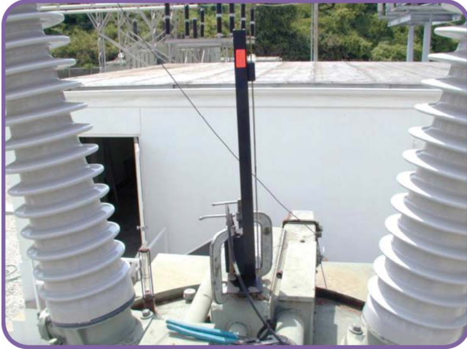
Figure 26. Linear Transducer on an OCB
