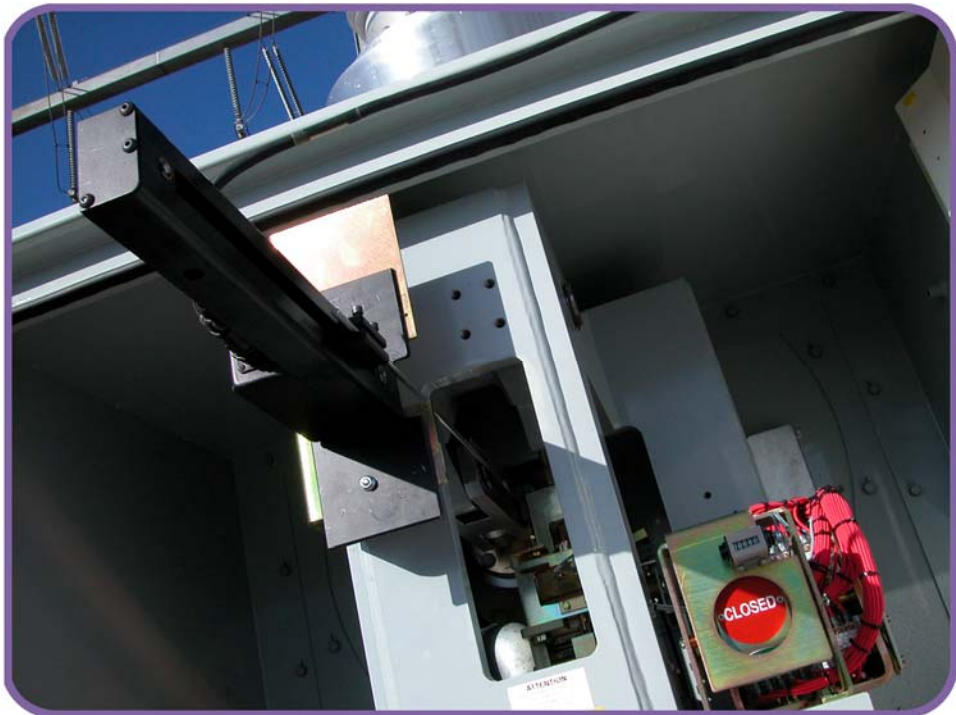
Figure 33. Linear Transducer on Mitsubishi 500-SFMT
