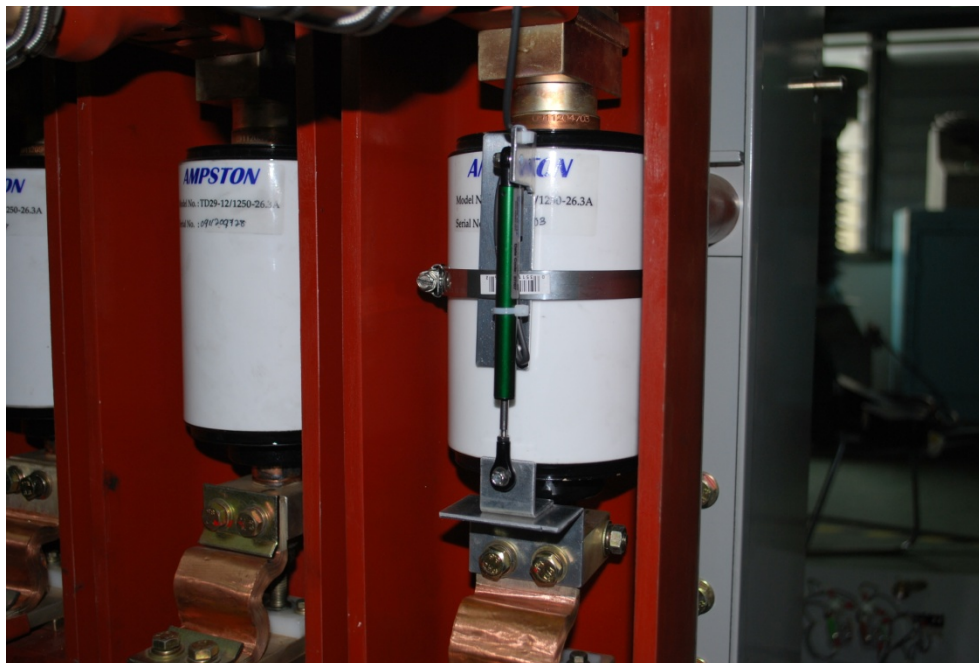
Resistor Transducer on Vacuum Circuit Breaker
